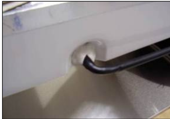
Figure 19: Drain pipe and putty
