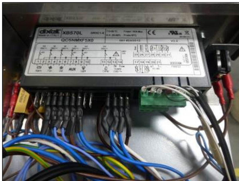
Figure 26: Wiring connections to XB570L controller
